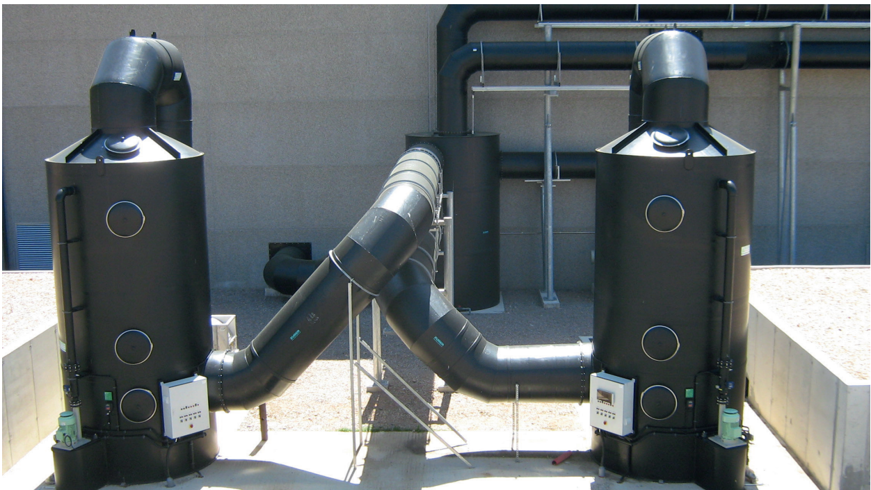
Immersible pumps on scrubbers
