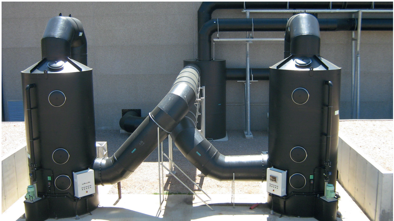
Immersible pumps on scrubbers
