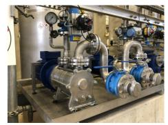
SCE MAG-M65, for pumping of ISOBUTYLENE Q=35 mc/h, H= 40m; Ningbo - China.
