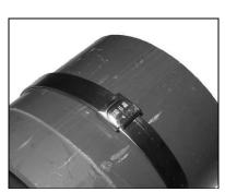
**9.** Complete clamp by tapping lip of band over buckle and remove ratchet wrench from tool as shown in step 6.
