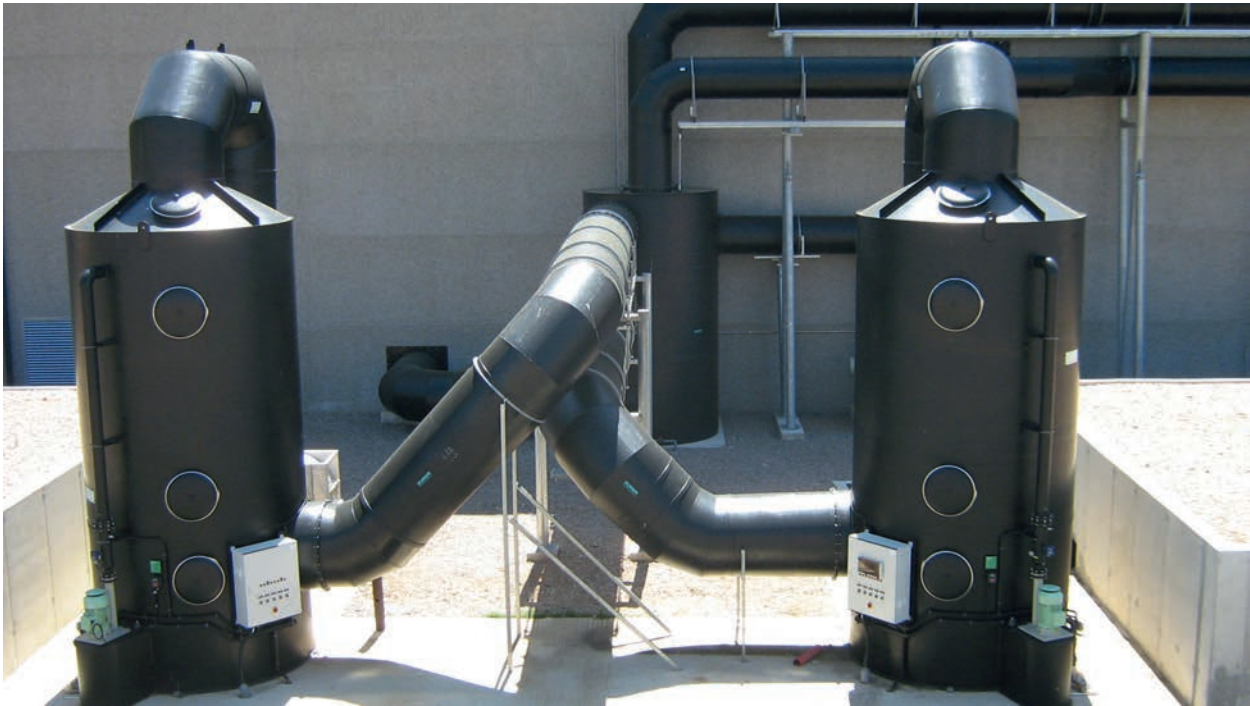
Immersible pumps on scrubbers
